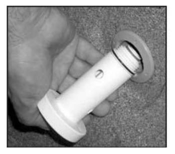
3. Remove jet wrench and jet internal nozzle assembly. Inspect condition and lubricate 0-rings as needed.
