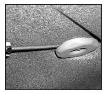
1. Insert a flat screwdriver between the jet face and the spa shell. Twist the screwdriver to pop the jet face.
